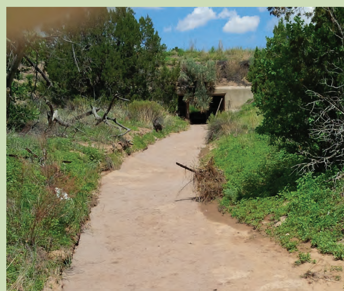
Storm flow in typical ephemeral channel
