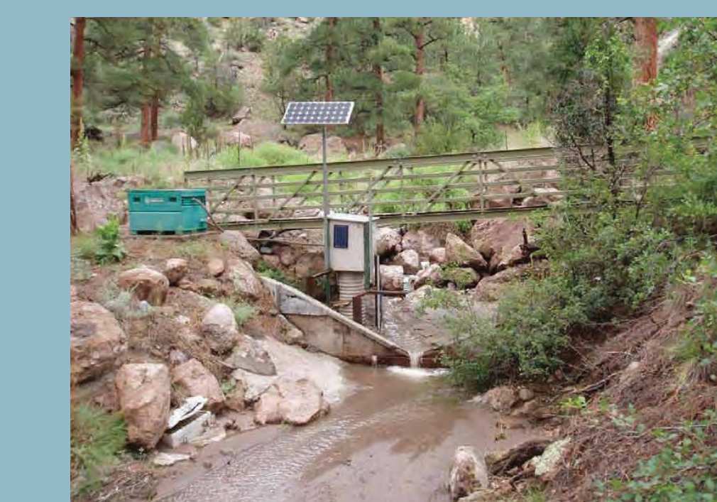
Typical surface water monitoring gage station
